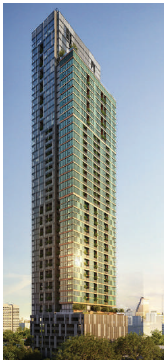
THE LOFTS SILOM-MAIN TOWER
